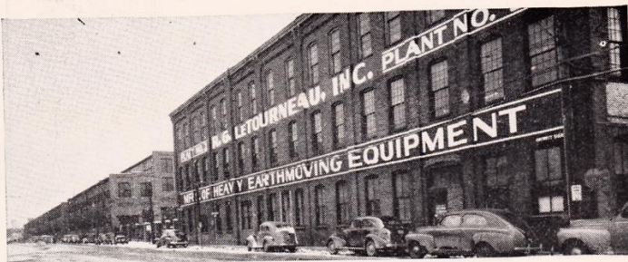
LE TOURNEAU INDUSTRIAL PLANT
