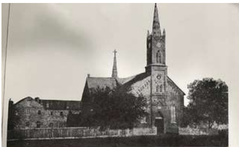
Church and monastery in about 1880. Note that front steeple is atop roof. In 1881 it was removed and rebuilt.
