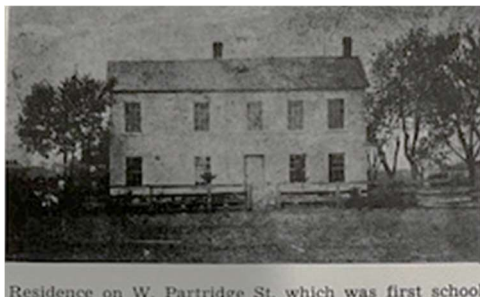
Residence on W. Partridge St. which was first school.
