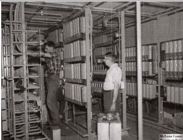
R.W. Rauh, president of the Metamora Telephone Company, watches the installation of the new dial apparatus in 1958
